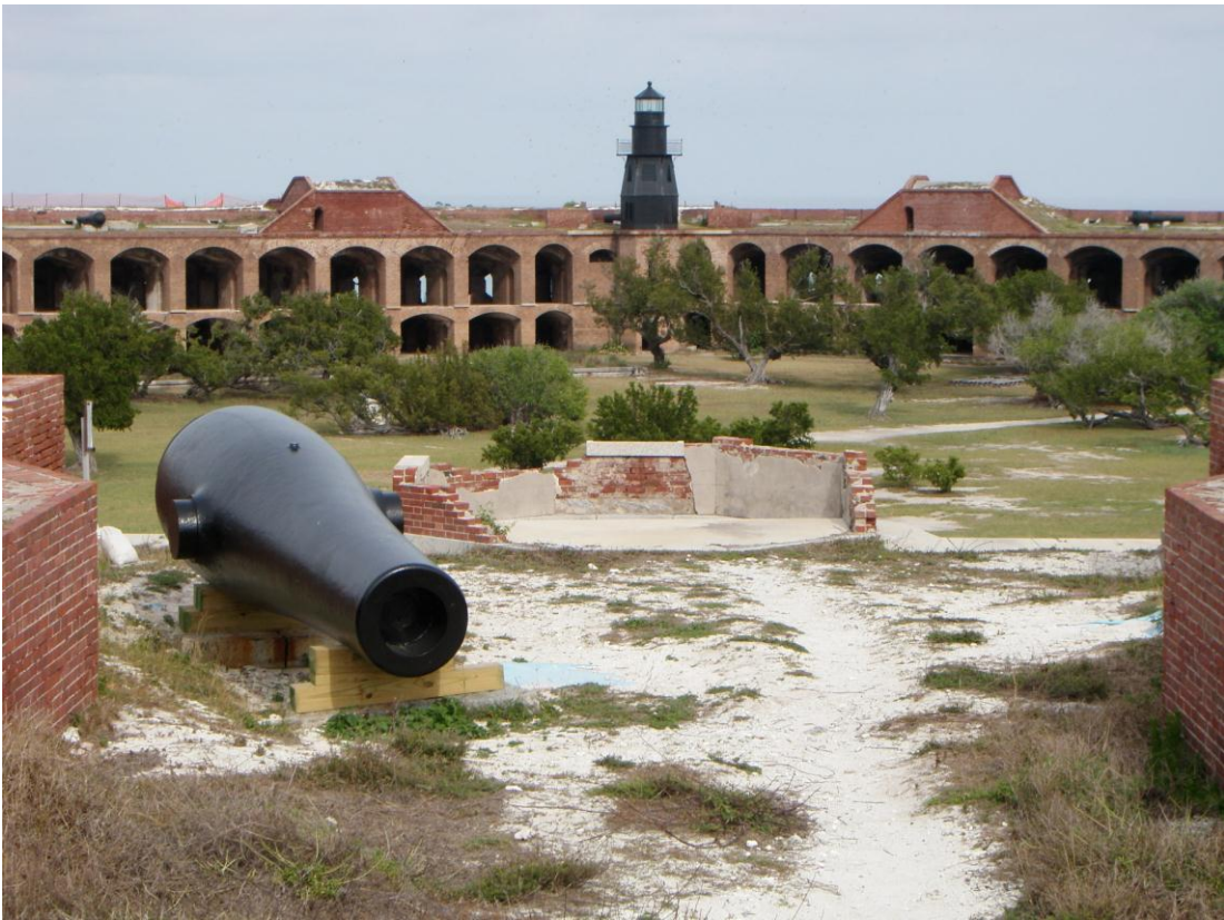
Looking in from the top
