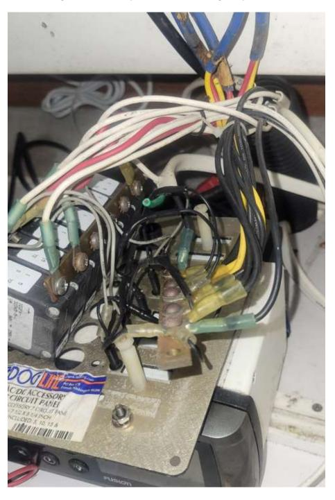
Rather than run longer wires to the breaker panel, I decided to minimize the wires going to the panel and use some bus bars and terminal blocks instead. Some other parts of the update:
