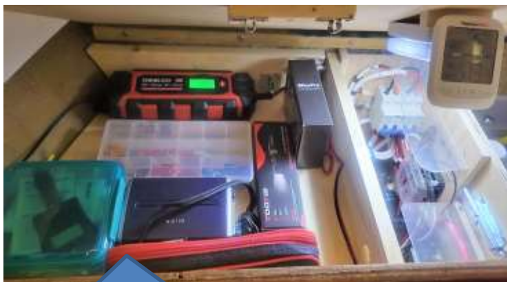
Charger in front with extra fuse container in the middle and small inverter (that can plug into lighter outlet) below that
