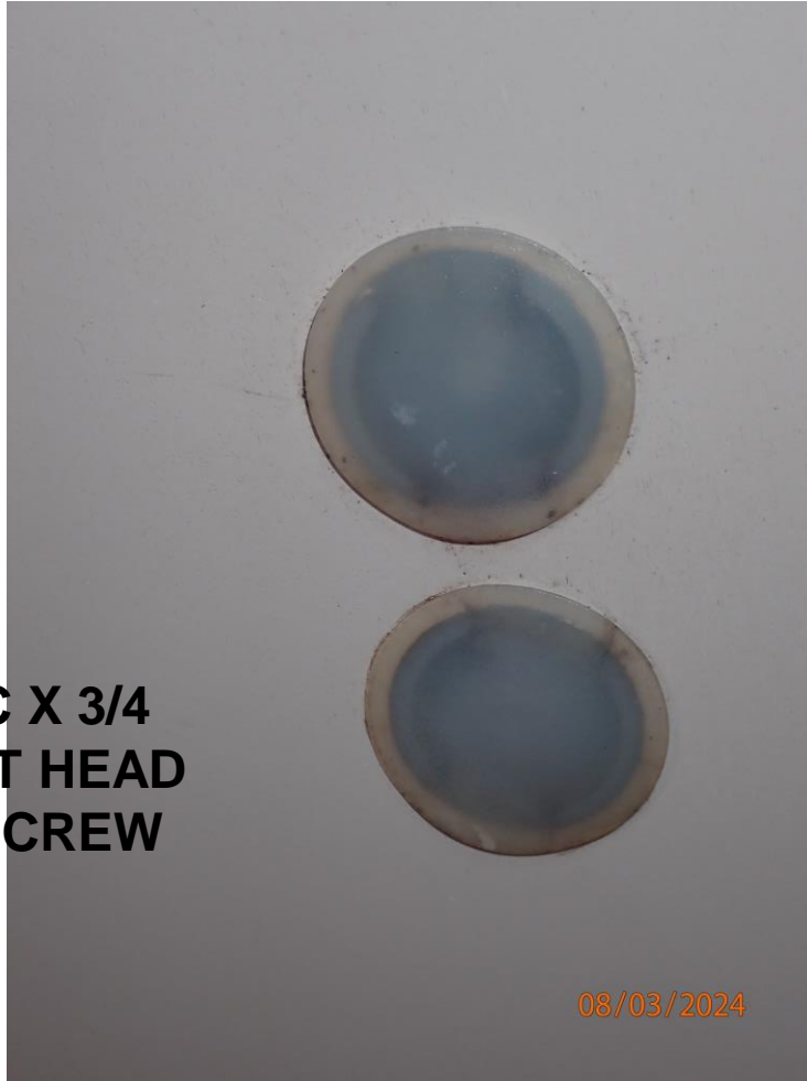
INTERIOR VIEW SHOWING SNAP-IN CAPS
