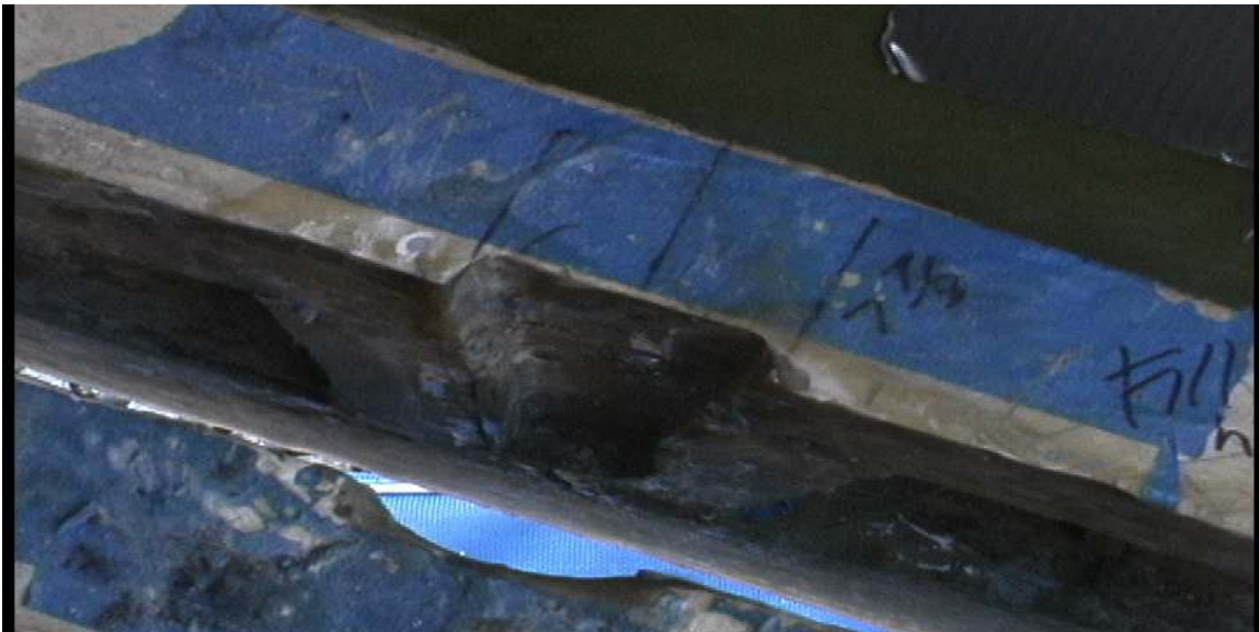
The pivot slots shown after they were taken out and restored
